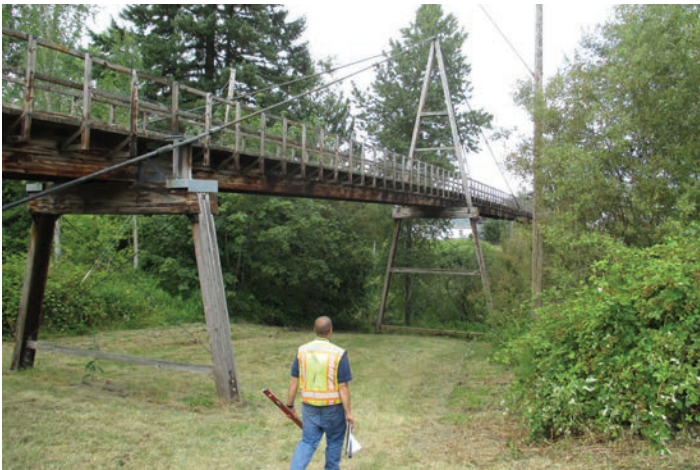
Jared inspecting the bridge in 2013.
