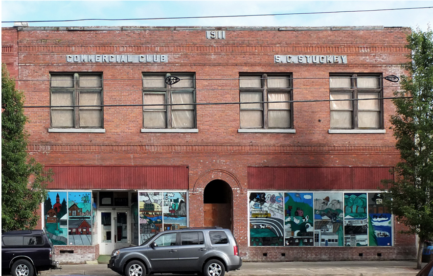
A contemporary image of the Stuckey Building
